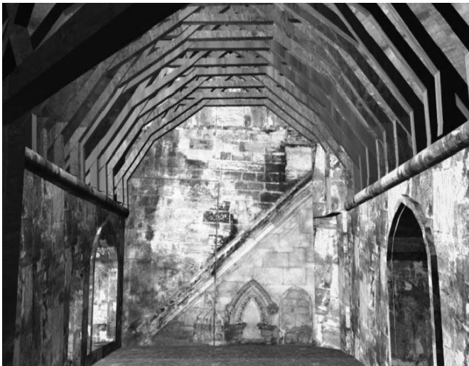
Fig. 4. Mason's Loft – North Transept Wall.
