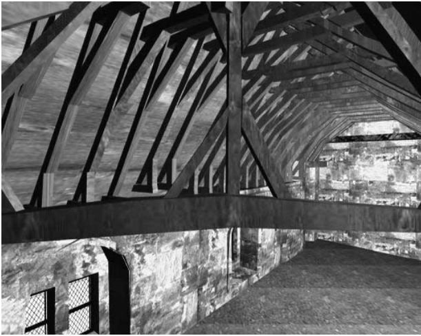
Fig. 3. Mason's Loft – Scissor-braced roof.
