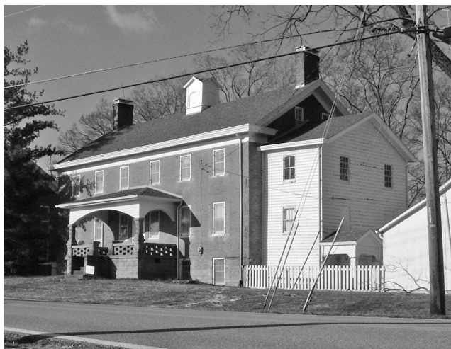
Figure 3. Dwelling House at present.
