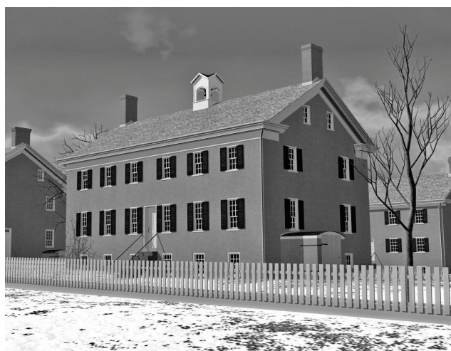
Figure 4. Dwelling House with 19th century configuration.
