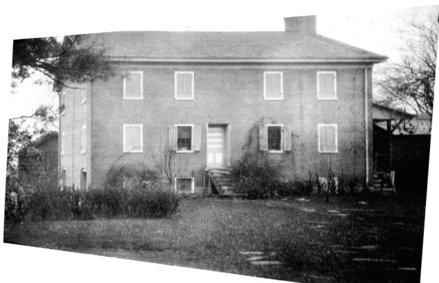
Figure 5. Sisters' Shop rectified photograph.
