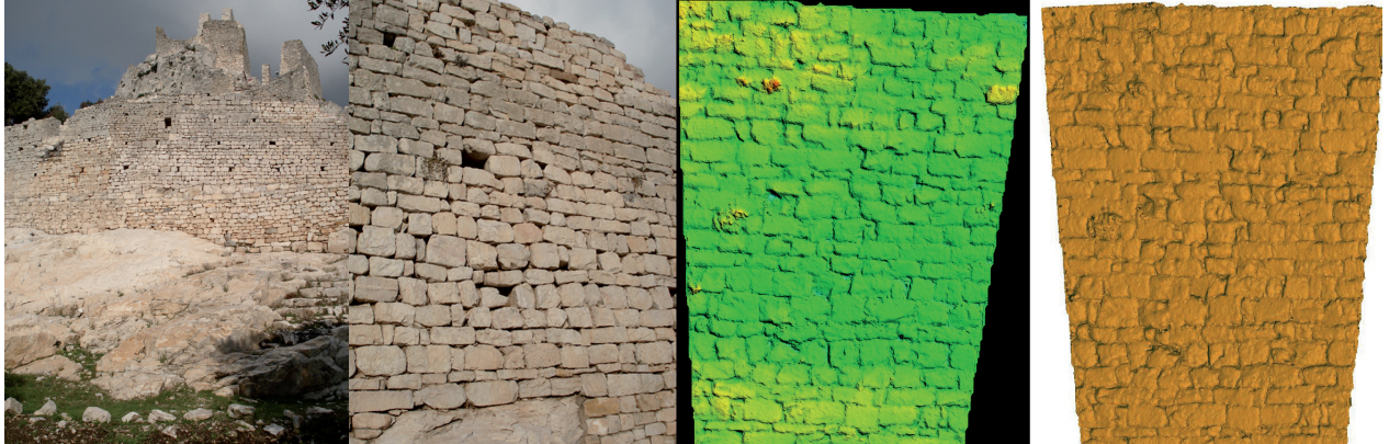
Fig. 3. S. Silvestro rock near Piombino (Italy) and the detailed 3D modeling of its rock walls, simply from 3 convergent images acquired with a consumer grade digital camera with 6 Mega pixels.
