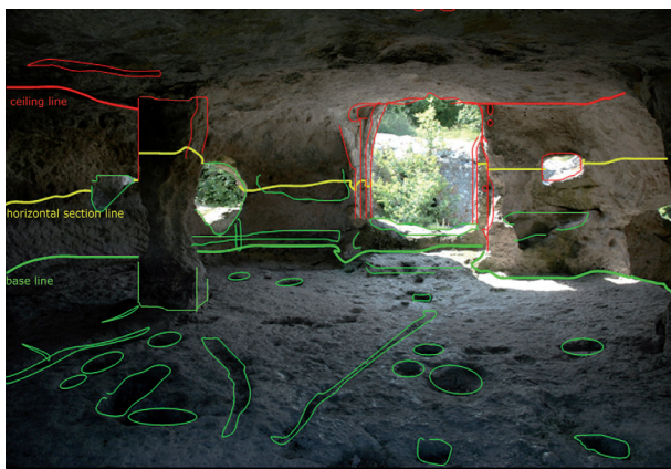
Fig. 4. The measuring of carved objects in a cave considering the position below (green) or above (red) the section line.
