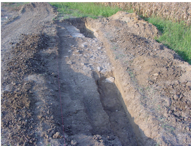
Fig. 3. Excavation cutting. Via Egnatia. (Karadedos and Nikolaidou 2007).
