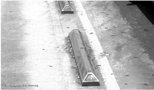
Figure 17: Lane separator blocks (Source: FJELLSTROM, ITDP 2007).
