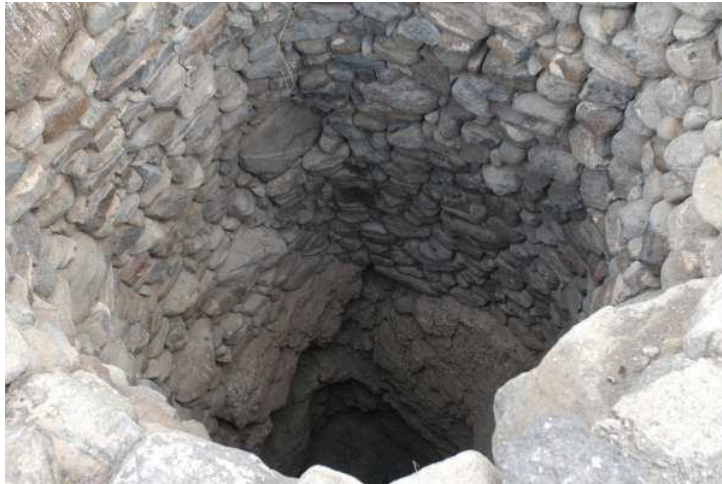
Figure 4.5: Masoned well shaft south of the archaeological site HLO1. The shaft is preserved to a depth of about 10 to 15 m.
