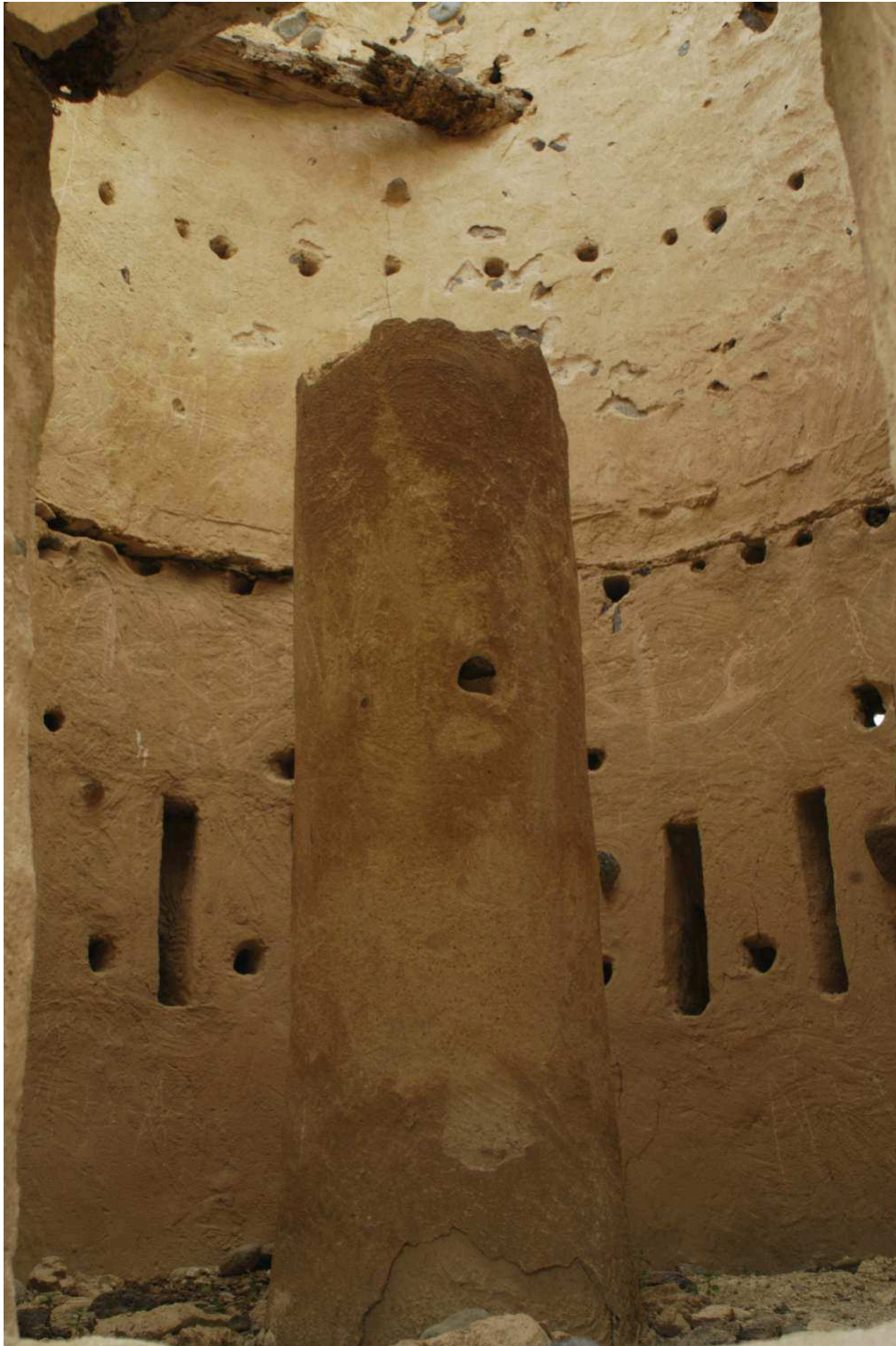
Figure 5.65: Column inside the modern tower.
