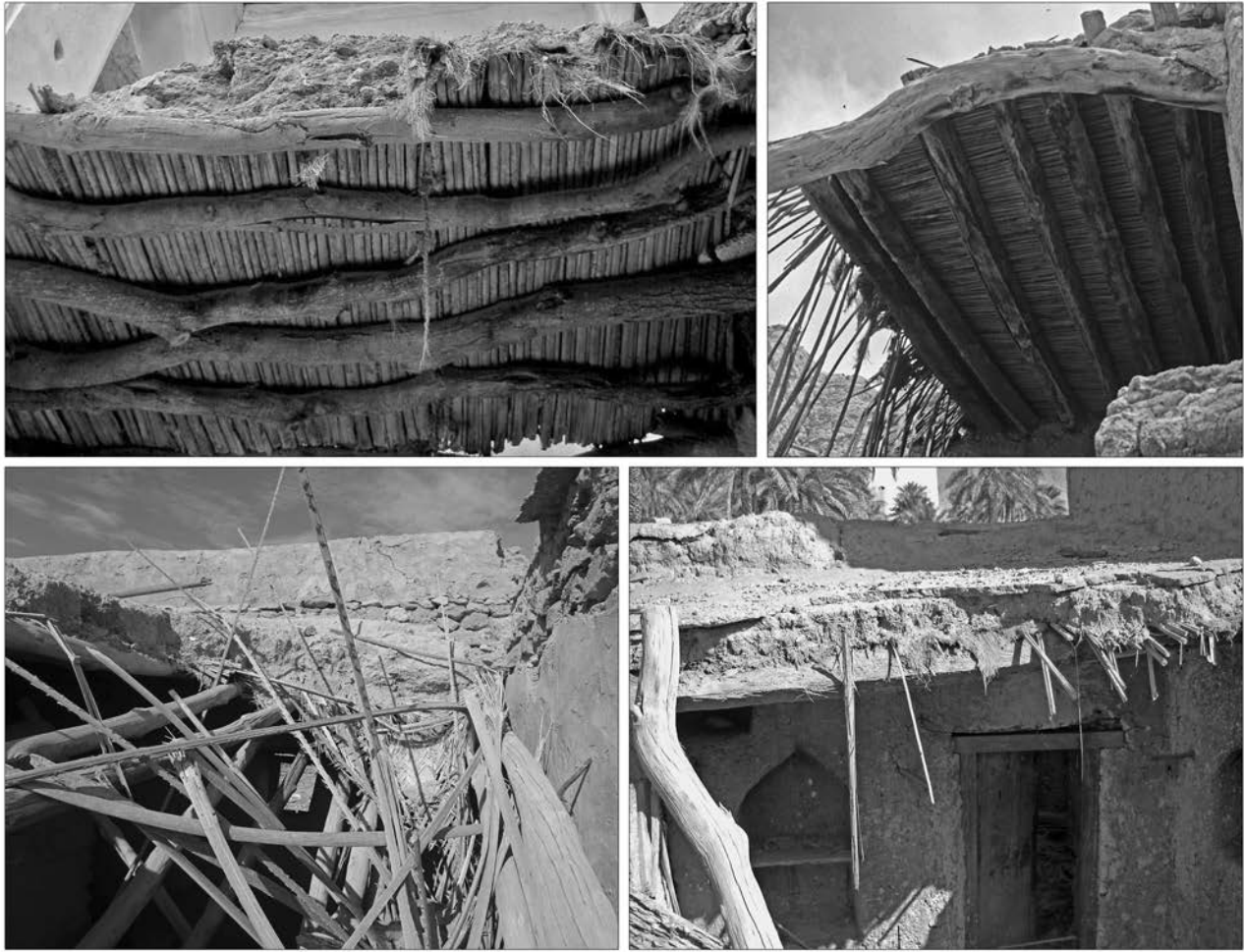
Fig. 9: Examples of roofs built with wood beams, mats and earth, typical of regional architecture (Photos: V. Azzarà, top right S. Cleuziou).
