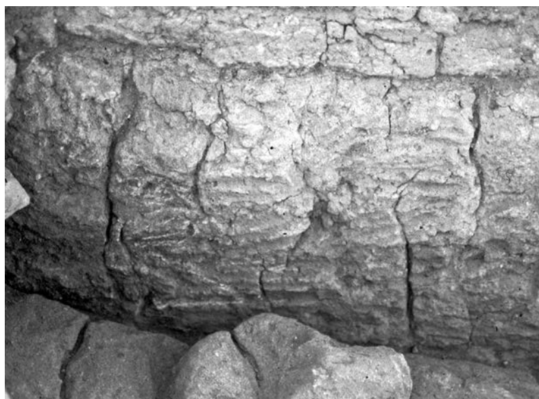
Fig. 11: Plastering with finger marks preserved in Room 13 of Building II (Photo: JHP).
