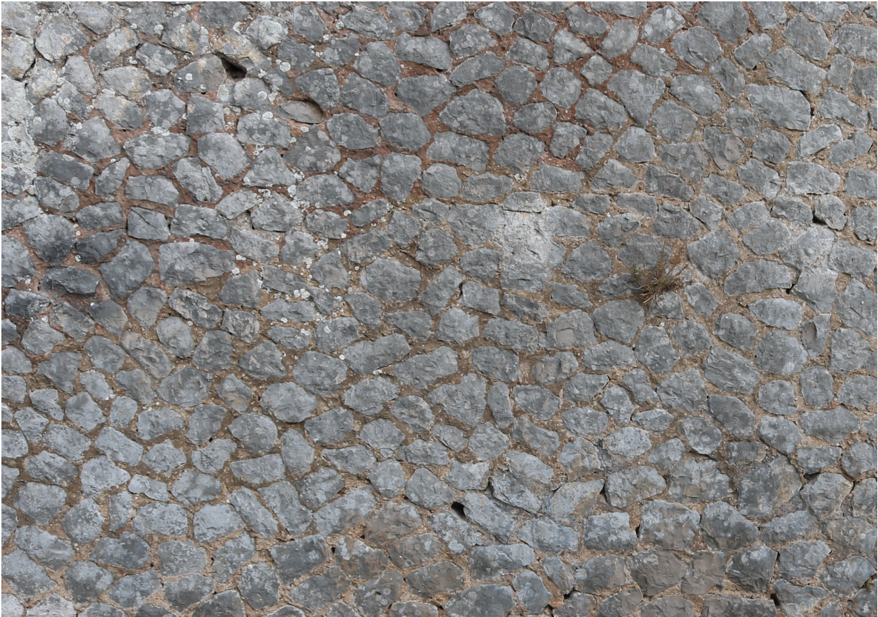
Fig. 6. Opus incertum facing from the sanctuary of Terracina in Latium (early 1st cent. BC) (photo by D. Maschek).
