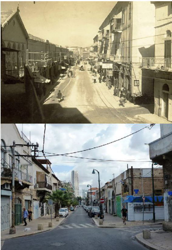
Figure 11: The Entrance to Bustrus Street. Photograph from the 1920s, taken from the Howard section of the street, and the same site photographed in 2018. Source: Private archive of Samuel Giler.
