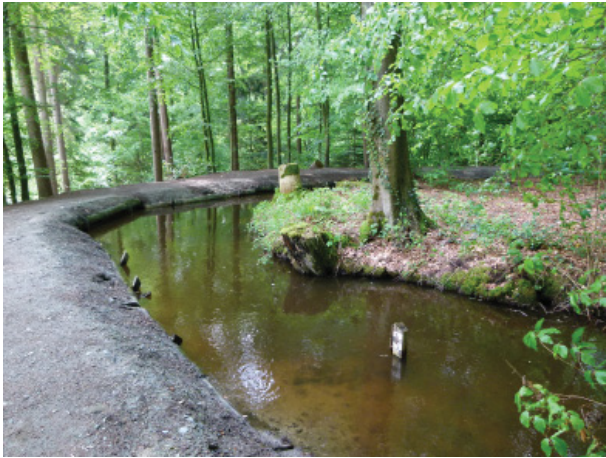
Fig. 6. The ‘silent stream’ of Weingarten. The construction parallel to the hillside made it possible to control its speed (Photo by Christina Vossler-Wolf).
