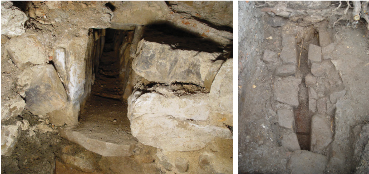
Fig. 4. Bebenhausen. Water channels in the cloister around 1200 AD. Left: in the foundation of the cloister; right: under the foundations of the western wall (Photos by Christina Vossler-Wolf).
