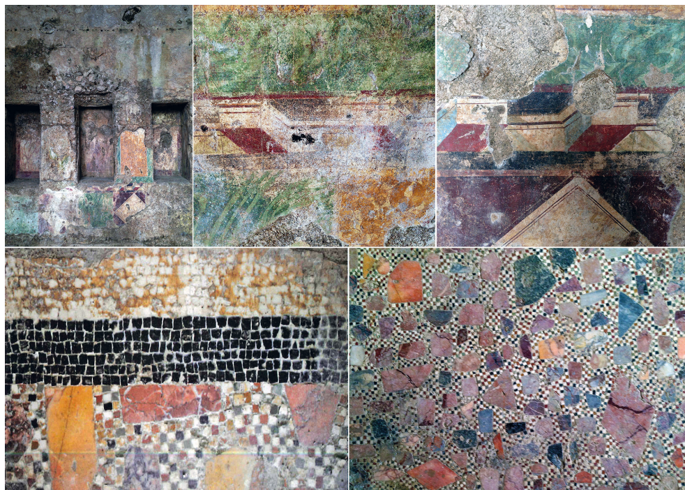
Figure 4. The rich decorative apparatus, wall and floor details: below the niches, is a pseudo-perspective representation of the architectural elements, colored red, white and blue; while the flooring mosaic system is formed by a three-colored tessellated floor with crustae marble, and a “rustic mosaic”.
